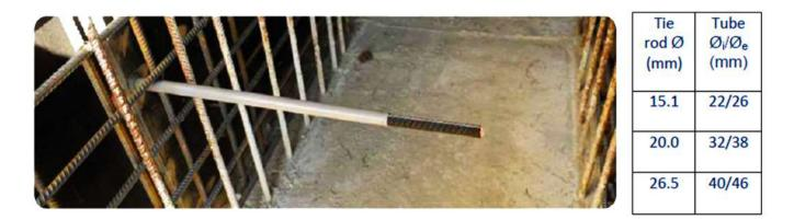
For passage of the tie rods through concrete walls.
